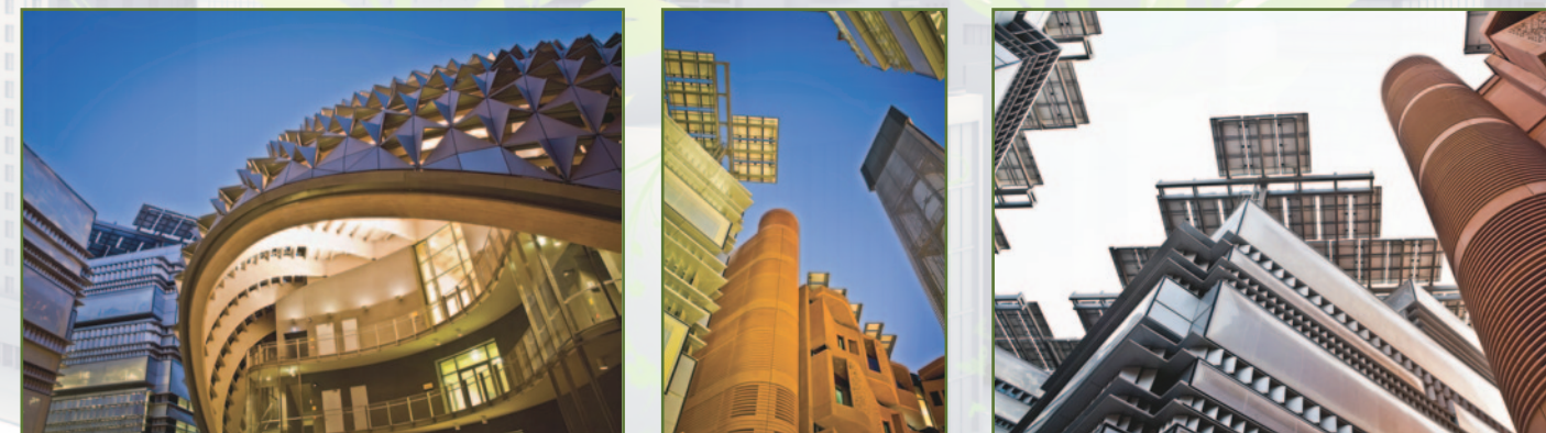
Various views of the Masdar Institute Building and the Knowledge Centre, Masdar City, UAE
