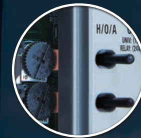
Potentiometers provide variable voltage to outputs in Hand
